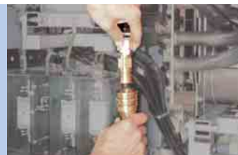
3. Liquid cooling can be disconnected quickly and without any spilling using quick couplings.
